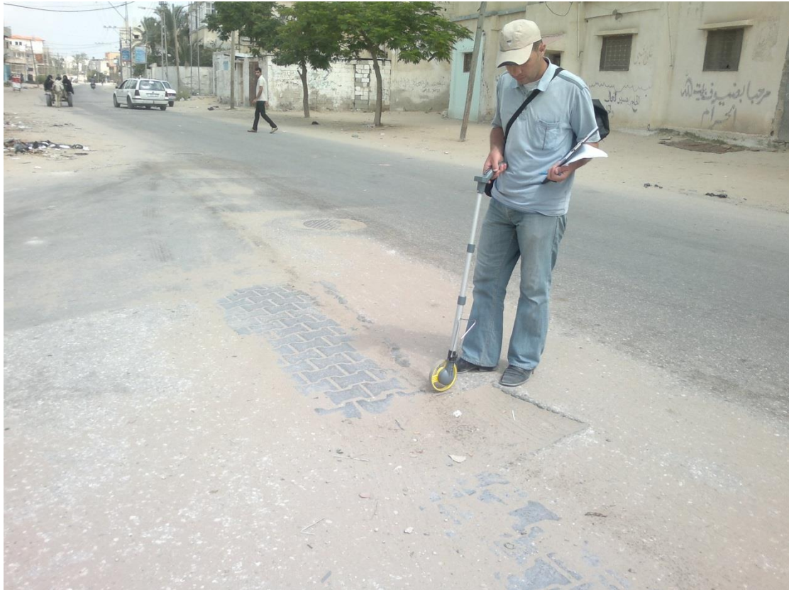
Figure (3.7): Pavement Condition inspection in Taha Hussien street.
